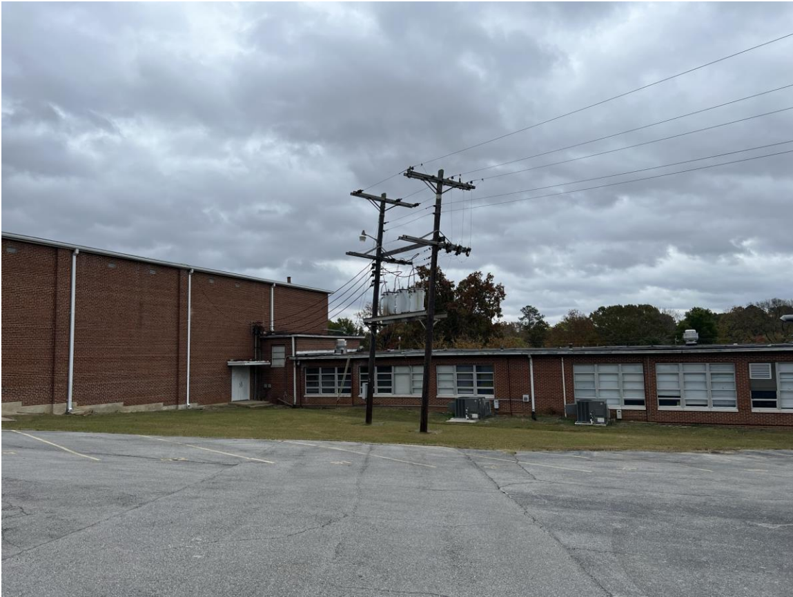
Leaning supports of Electrical transformers
