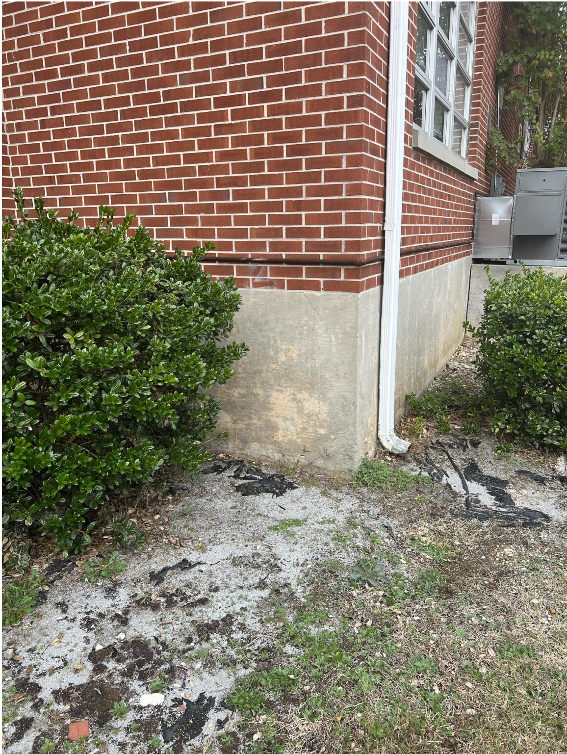
Vegetation close to building and downspouts draining onto grade
