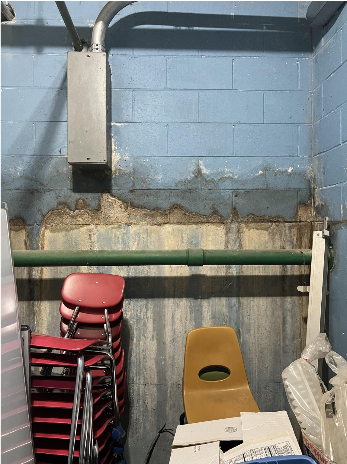
Water intrusion into Mechanical Basement
