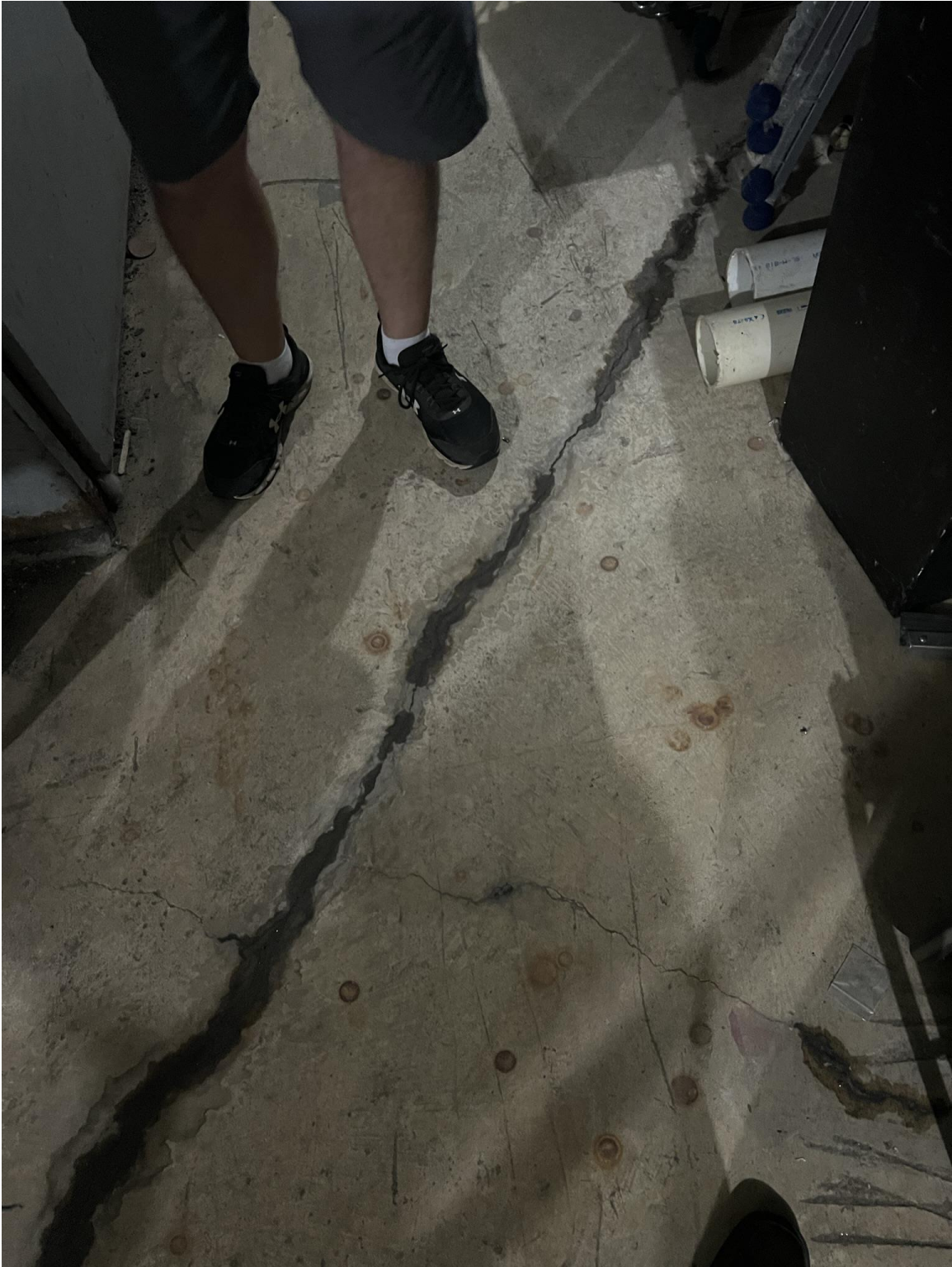
Water seeping up thru crack in basement floor
