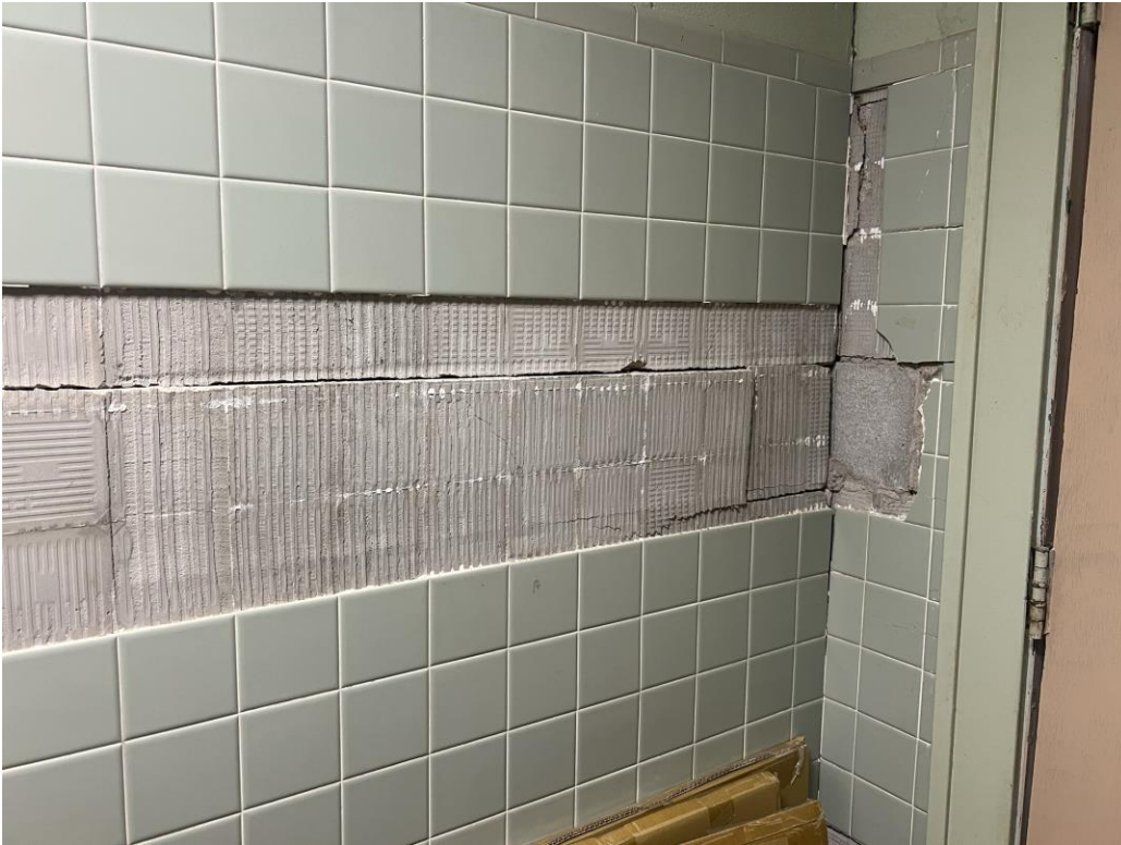
Cracking of the walls in the Storage Room adjacent to the Auditorium
