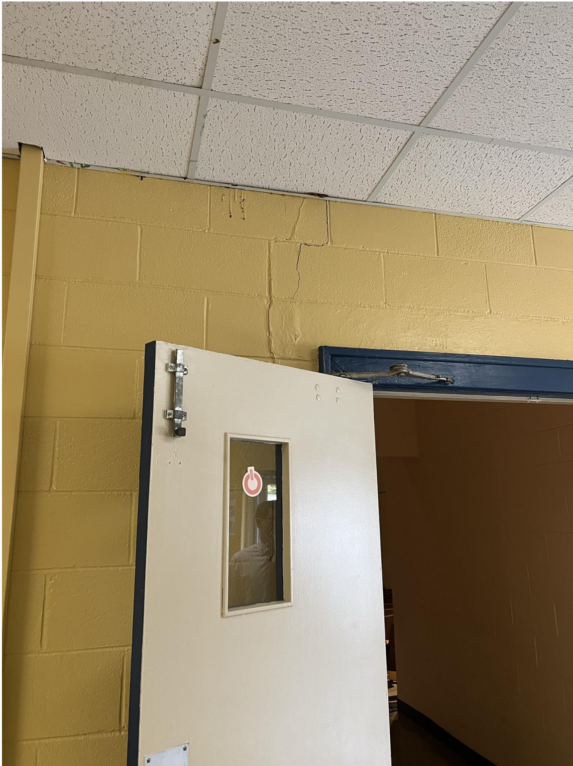
Cracking in interior masonry walls
