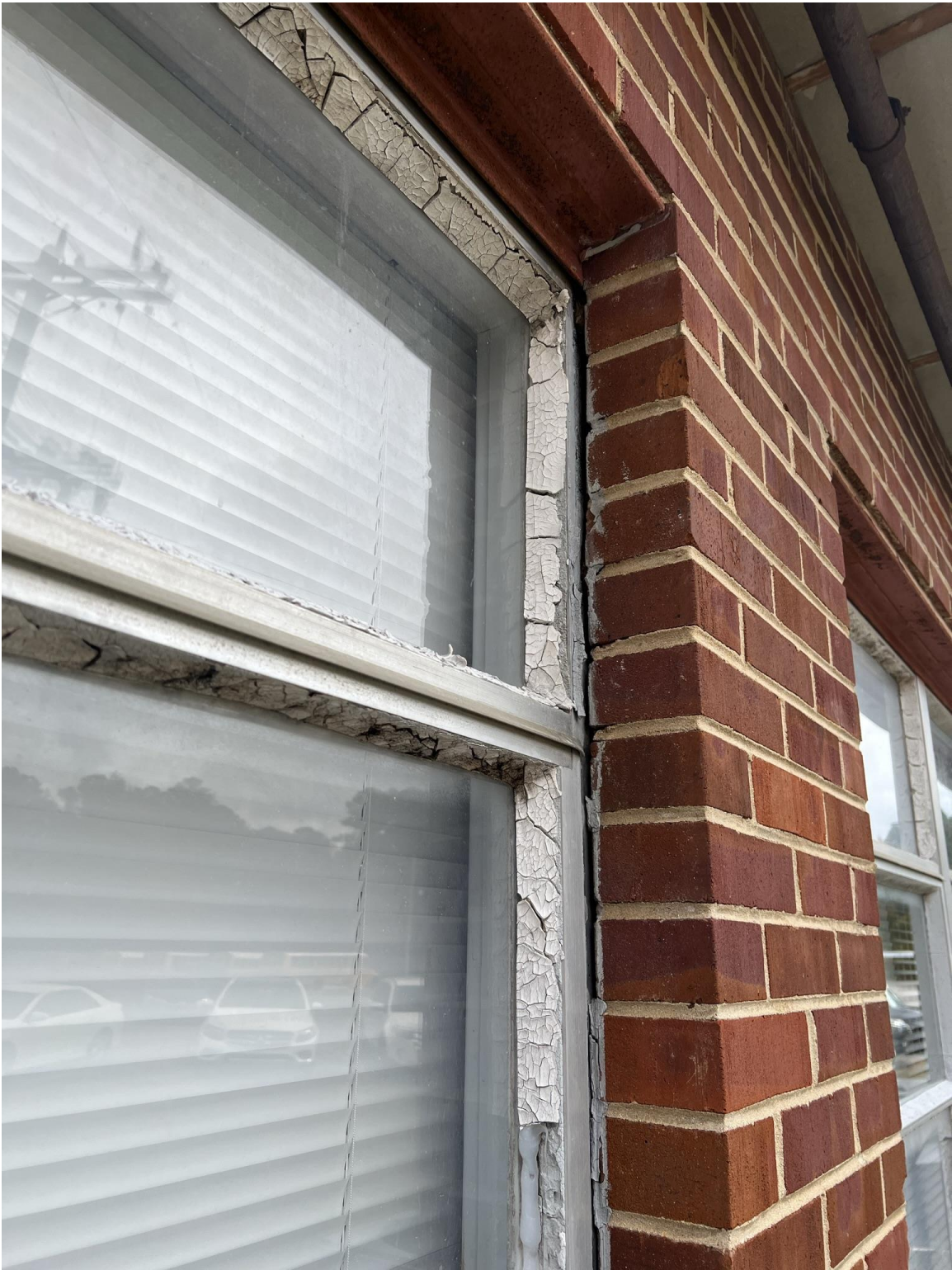
Windows separated at head and jambs
