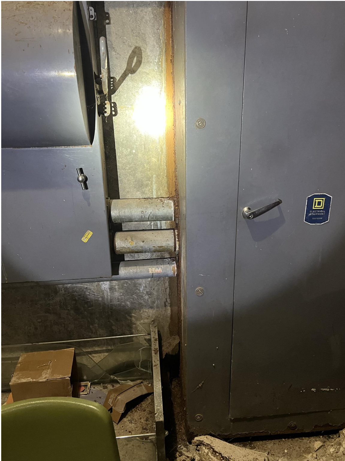
Water infiltration thru wall behind electrical panel
