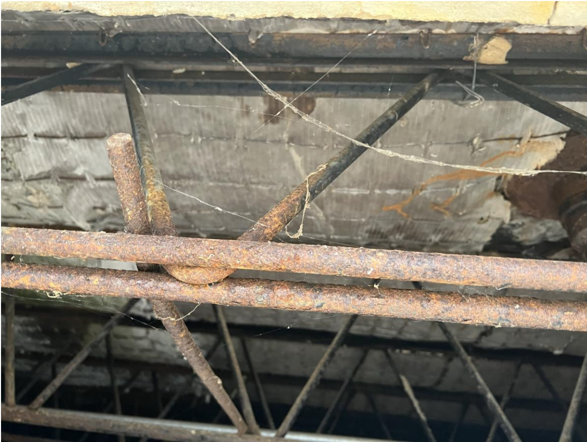
Rusting of bar joist floor supports at the Kitchen
