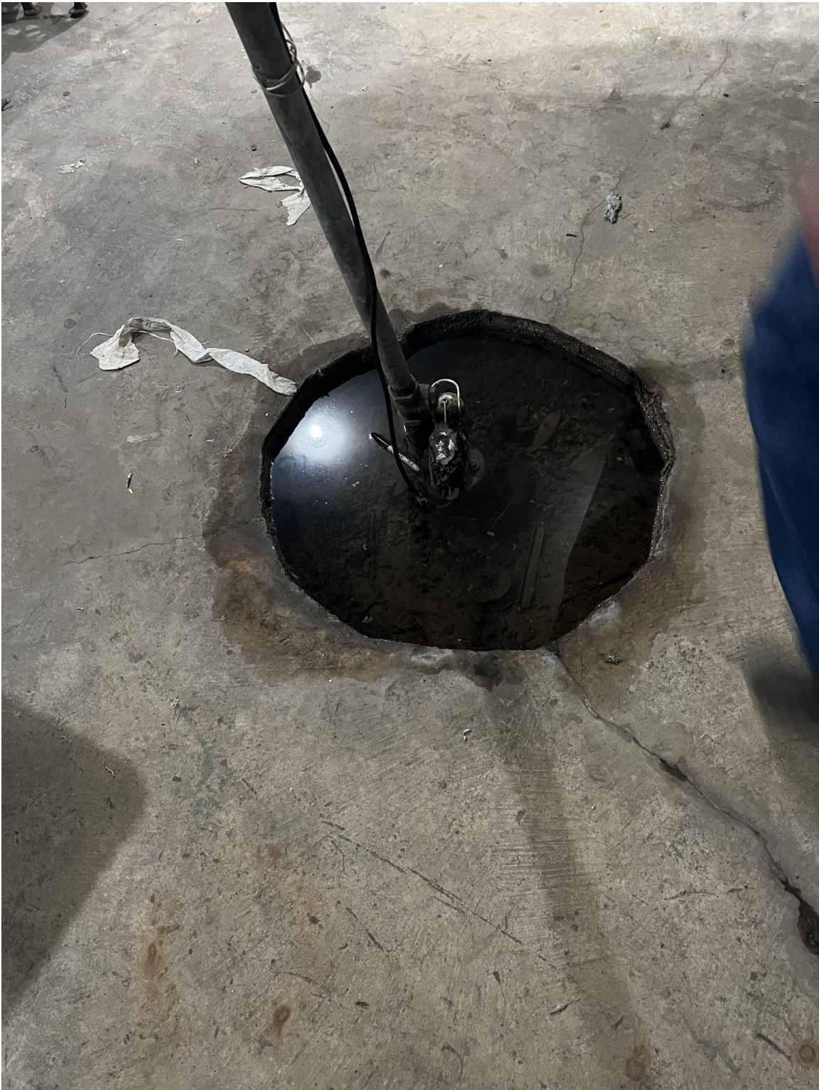
Sump pump is full and running continuously
